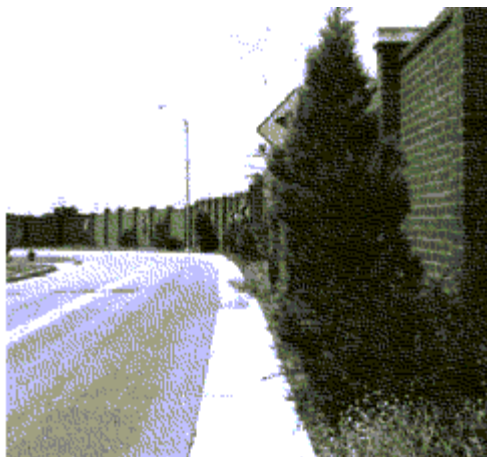
Brick Noise Barrier Wall FIG. 4
