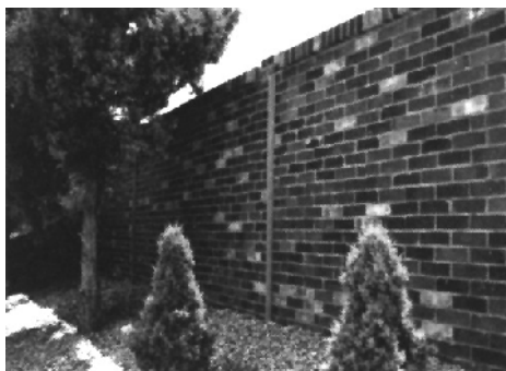
Steel Pier and Panel Wall FIG. 14
