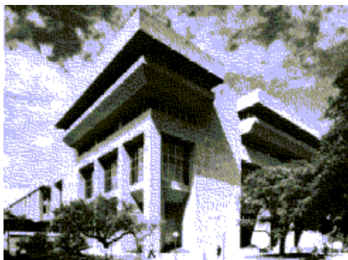
Evans Library, Texas A&M University - College Station, Texas
