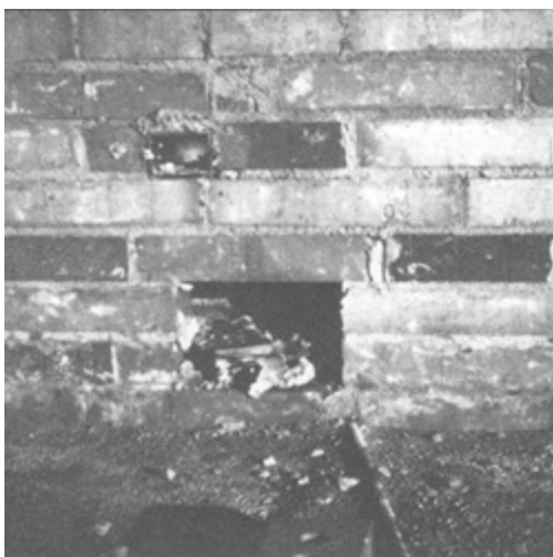
Grout Cleanouts Fig. 17
