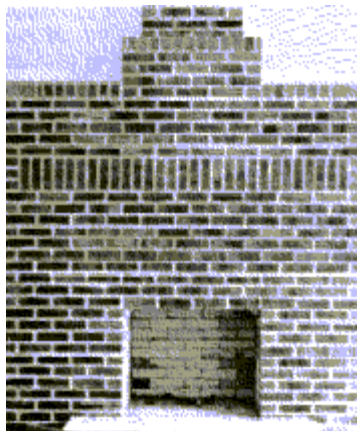
Contemporary-Style Brick Masonry Heater
