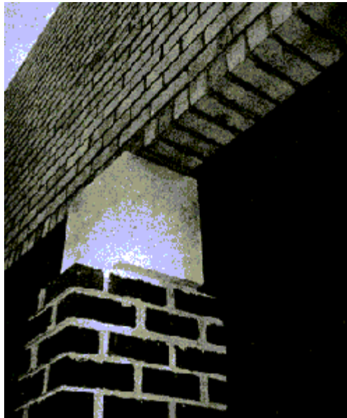
RBM Girder as Structural Facade - Maryland City Shopping Center
