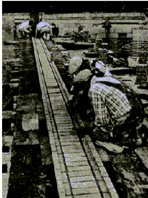
Soffit Brick in Place on Scaffold
