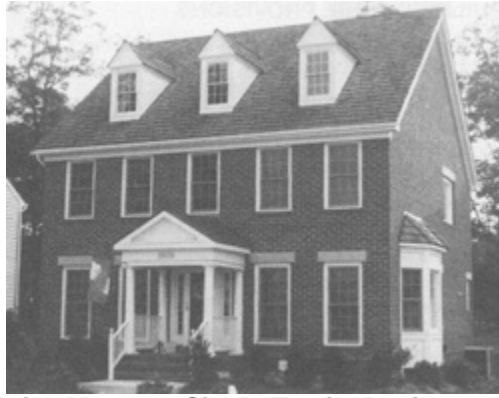
Reinforced Brick Masonry Single Family Residence, Ashbrun VA FIG. 6
