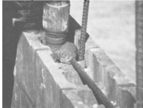
Reinforced Hollow Brick Masonry FIG. 4
